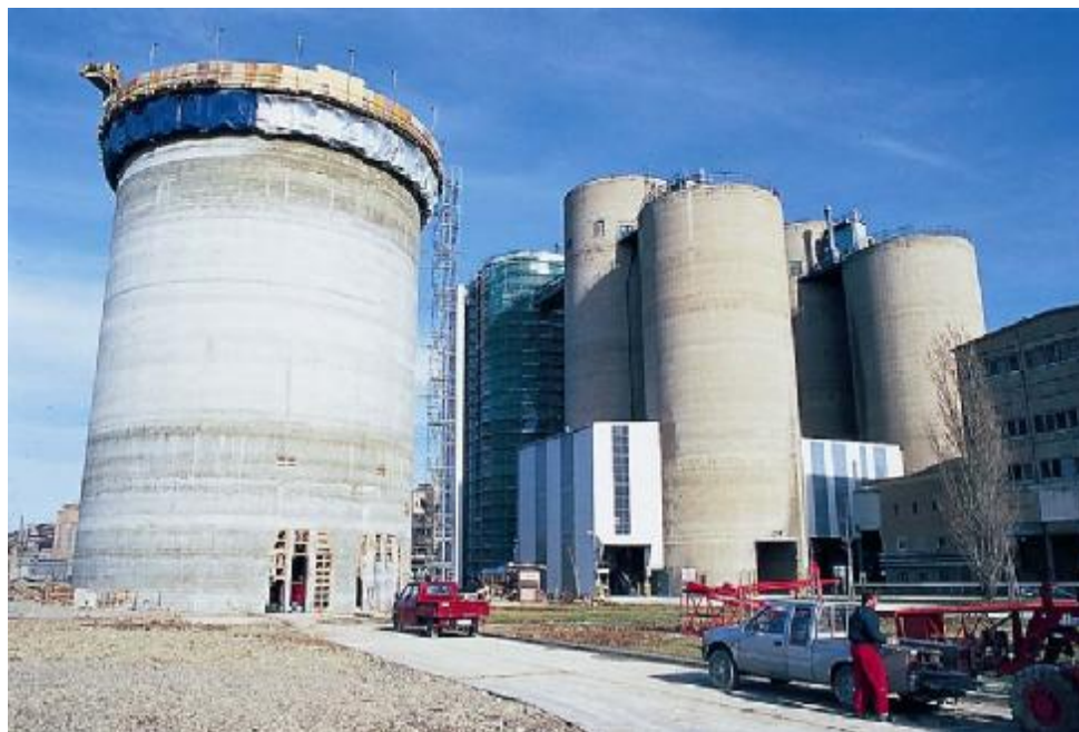
Fig. 7: Slipforming of a cement silo (Source: Peter & Lochner)
